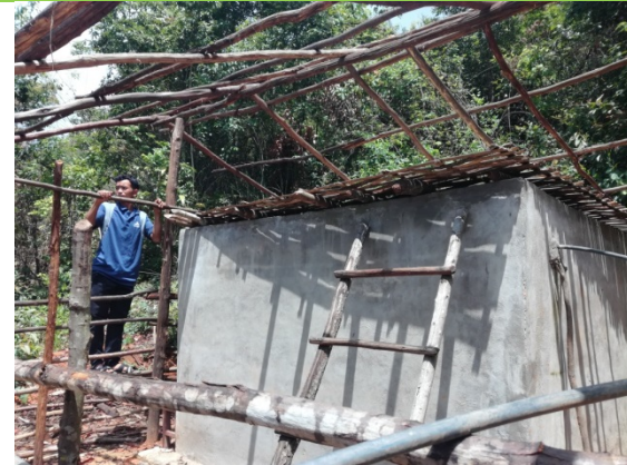
Figure 8 : water tank to supply water for livestock and for vegetables garden downstream
