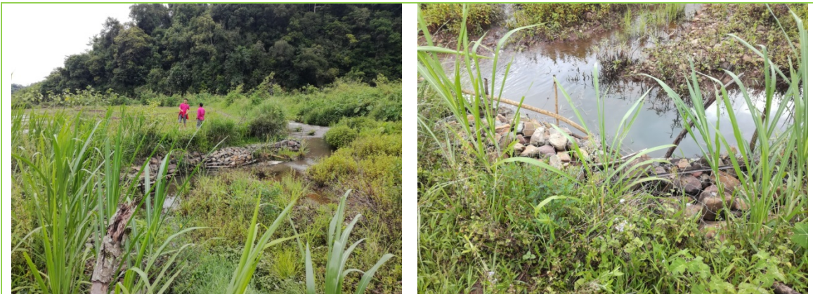
Figure 1 : Paddy bank reinforcement with gabion
